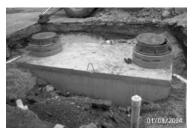
Grease Trap (under the sink & floor units)- make sure flow restrictor installed and properly vented.
